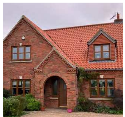
Figure 08: The images overleaf illustrate the common characteristics of Swinderby's built form: Materiality: red brick, render, stone, mottled brick. Detailing: Flemish bond, ventilation bricks, brick banding, decorative bargeboards. Roofscape: traditional pitch with bookend chimneys, hipped roofs and gablets, traditional pitch, catslide roof.
