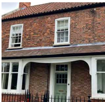
Figure 08: The images overleaf illustrate the common characteristics of Swinderby's built form: Materiality: red brick, render, stone, mottled brick. Detailing: Flemish bond, ventilation bricks, brick banding, decorative bargeboards. Roofscape: traditional pitch with bookend chimneys, hipped roofs and gablets, traditional pitch, catslide roof.
