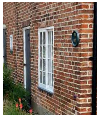
Figure 06: The imagery above illustrates the typical materials and colours on Swinderby's listed buildings. They typically include red brick elevational treatments, sashed windows, clay pantile roof tiling and brick banding.
