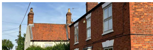
Stone / Wood Lintels and Sills
