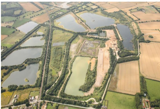
Aerial shot of Whisby Quarry
